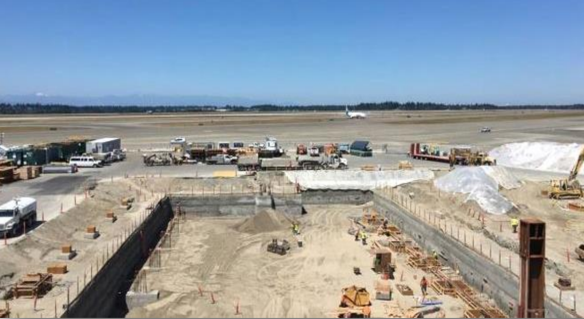
Expansion Excavation Area
