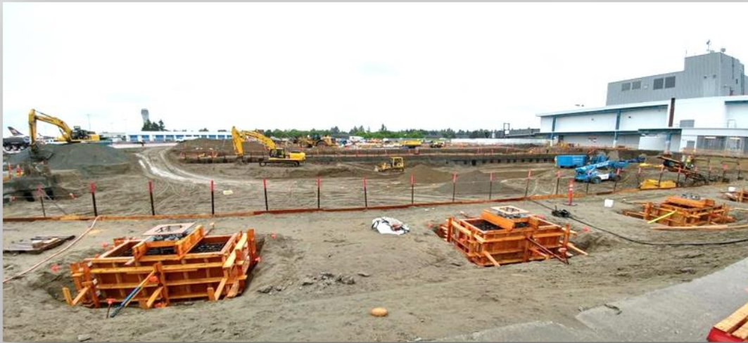
Excavation / foundation columns
